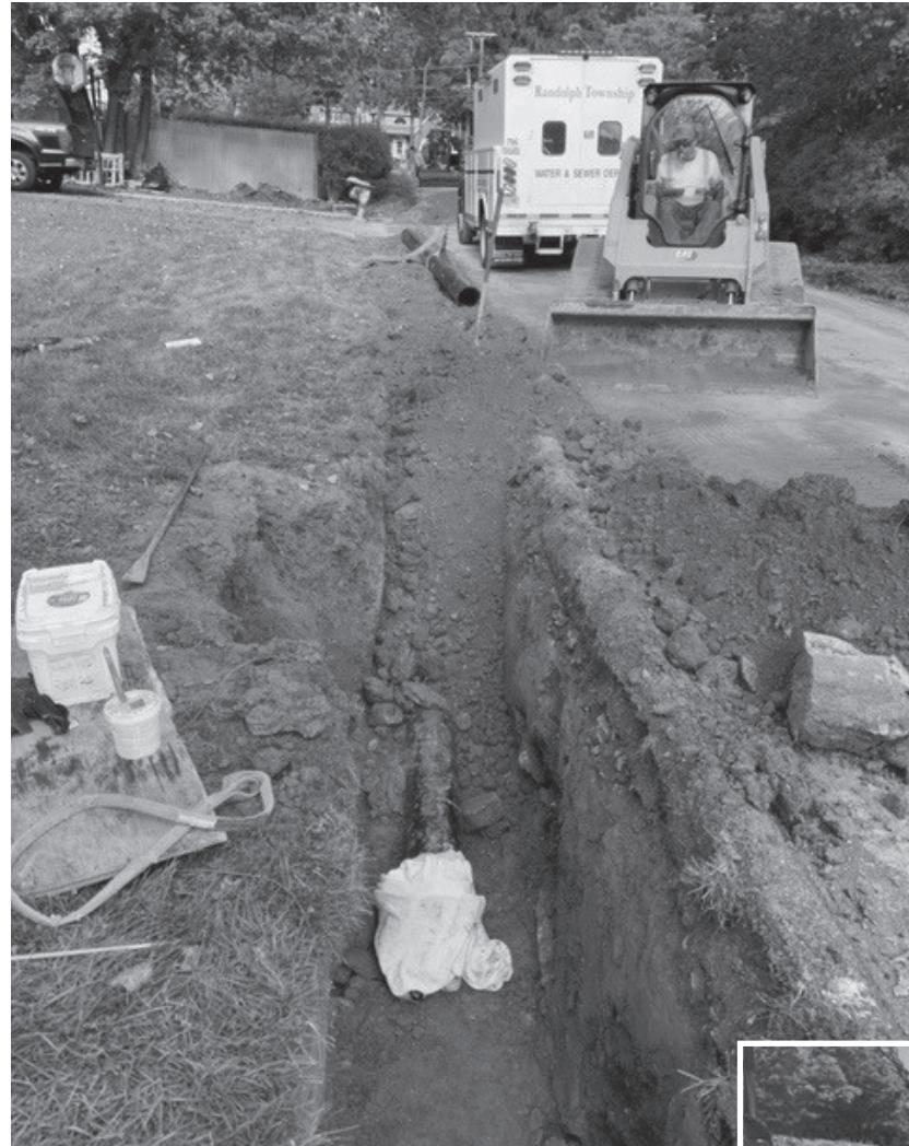
In October, the township's Water & Sewer and DPW staff installed a water main and fire hydrant along Birchwood Road. This new fire hydrant is necessary to improve fire protection for this neighborhood. This project will not include any new water services to residents at this time. All disturbed areas will be fully restored in the spring 2024.
