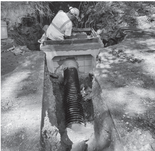
Doug Doland finalizing cement work on a new storm basin installed on the Combs Hollow drainage project.
