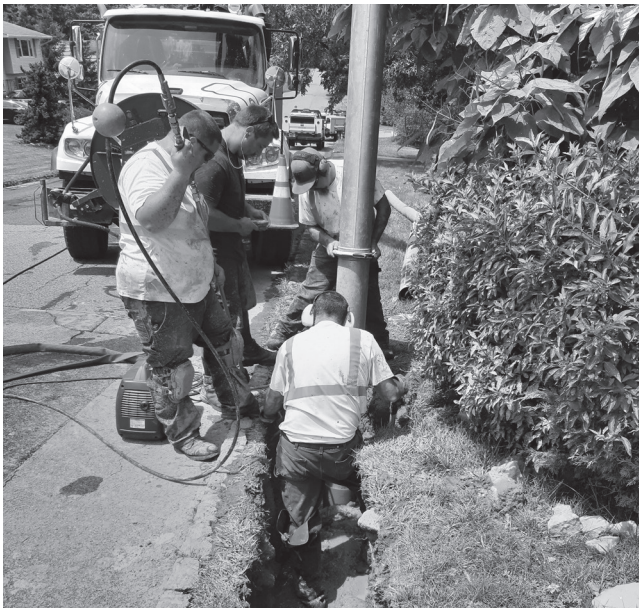
Tyler Muzzillo, Brett Fancera, Chuck DeCristoforo, and Robin Huff clearing a clogged pipe on the Rose Way drainage project.
