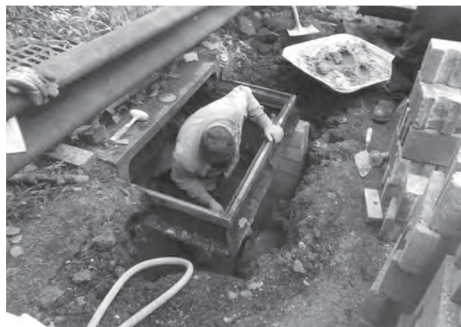
Township road crews at work – at left preparing Quaker Church Road for resurfacing, and at right rebuilding a stormwater catch basin.
