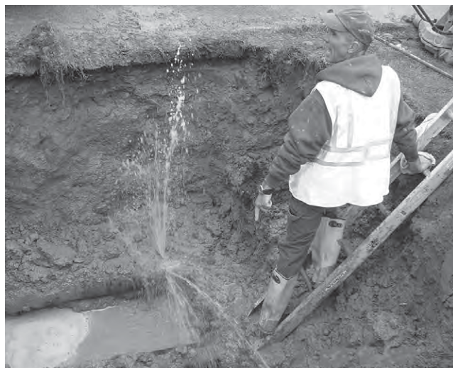
Water & Sewer Department crew working to repair broken water main.
