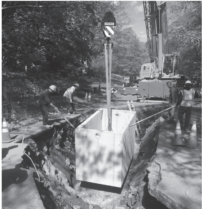
Water & Sewer Department crew works with contractor on an emergency repair to a water system pressure regulating valve on Deer Run Drive.
