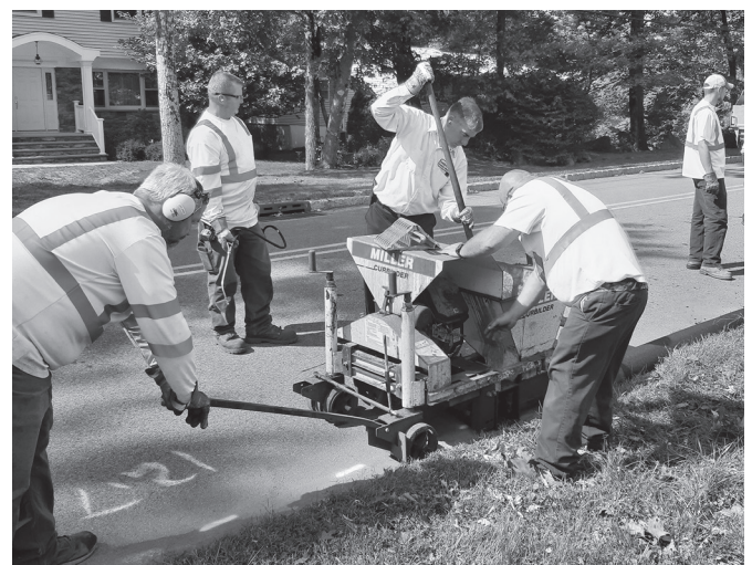
DPW crew installing a curb along Clover Lane.
