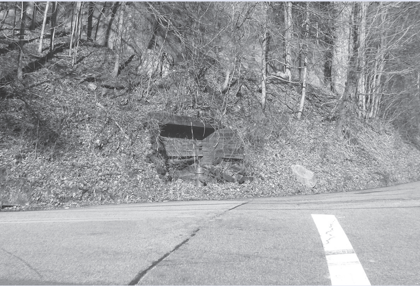
Deteriorated timber retaining wall at intersection of Millbrook Avenue and Fords Road – 1/6/2016.
