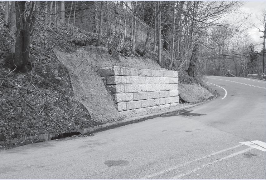
Replaced timber retaining wall with modular concrete block wall – 4/19/21.
